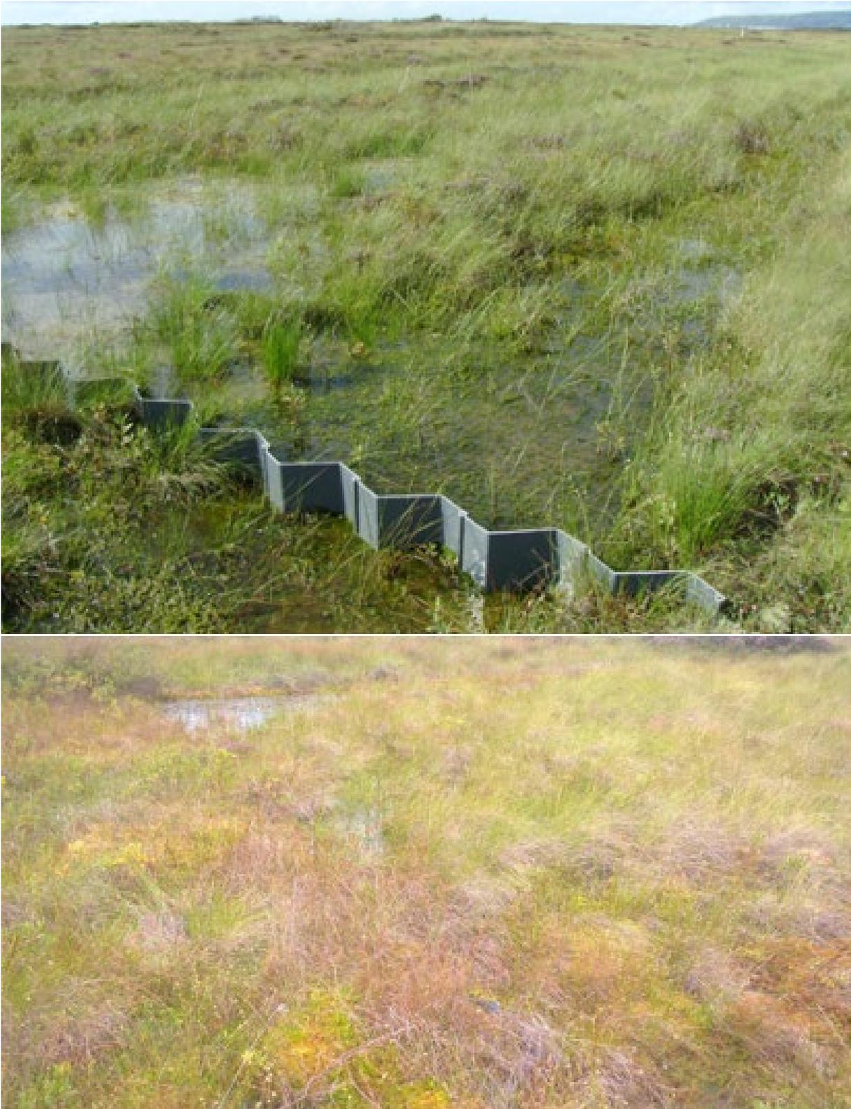
Figure 7. Above – Cutting one year after piling installed. Below – Cutting ten years after piling installed.
