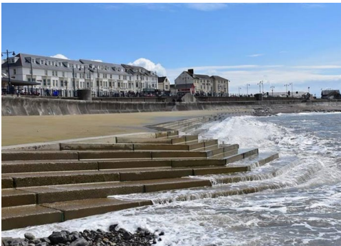
Figure 9 A terraced revetment Source: Porthcawl town beach re-opens to the public after £3m improvements to sea defences - News from Wales
