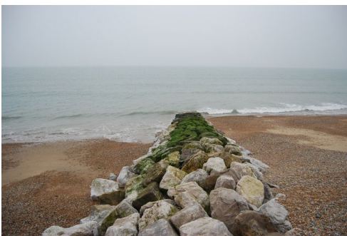
Figure 10 A rock groyne Source: Rock Groyne © N Chadwick cc-by-sa/2.0 :: Geograph Britain and Ireland
