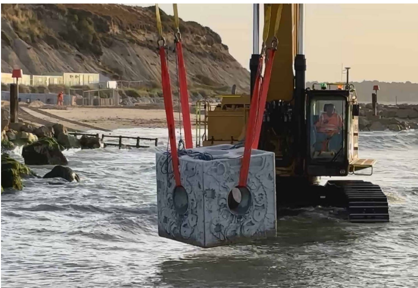
Figure 40 Installaion of ARC marine's low-carbon Reef cubes® (Source: ARC Marine)
