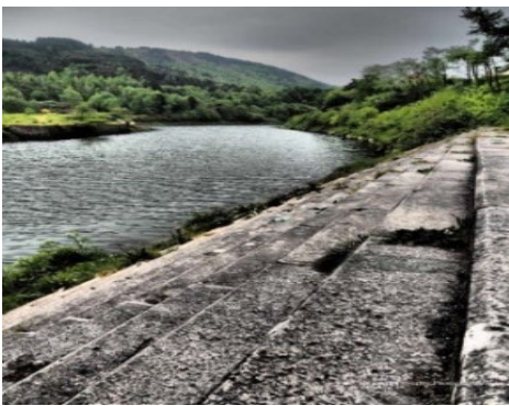
Figure 6 An embankment Source: River Tawe Swansea 2017 05 11 #28 | Gareth Lovering | Flickr
