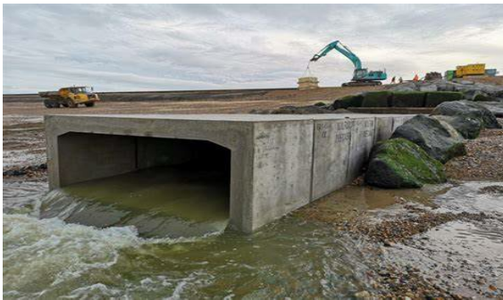
Figure 3 An outfall Source: Coldharbour outfall extension (2018) – Southeast Coastal Group (se-coastalgroup.org.uk)
