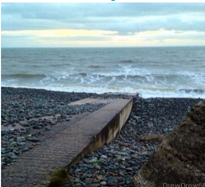
Figure 7 A ramp Source: We walked along to the concrete access ramp which enables ... | Flickr
