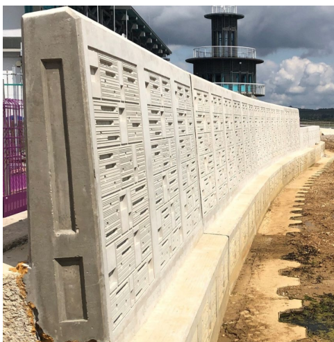
Figure 16 Technique 4 Cast-in textured, grooved and creviced concrete surfaces
