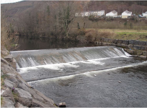
Figure 8 A weir Source: welsh weir - Bing
