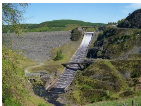
Figure 11 A spillway Source: Llyn Brianne Spillway | turbostar171 | Flickr
