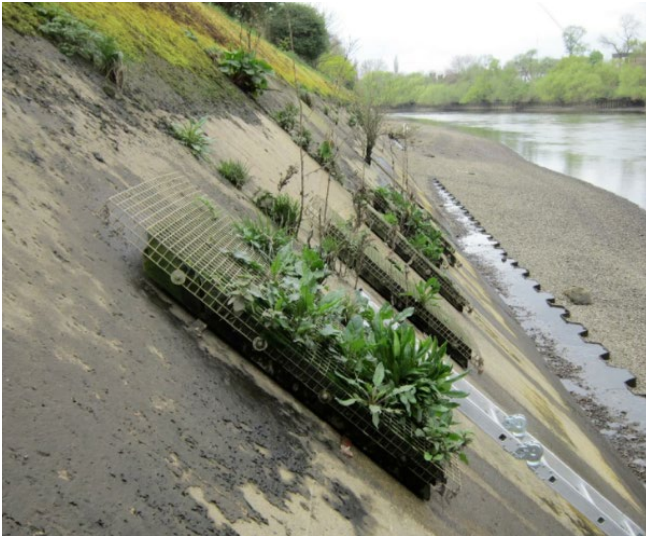
Figure 36 Vegetation cover at the wall modules at Kew Bridge Site (Source: Francis, R. 2015)
