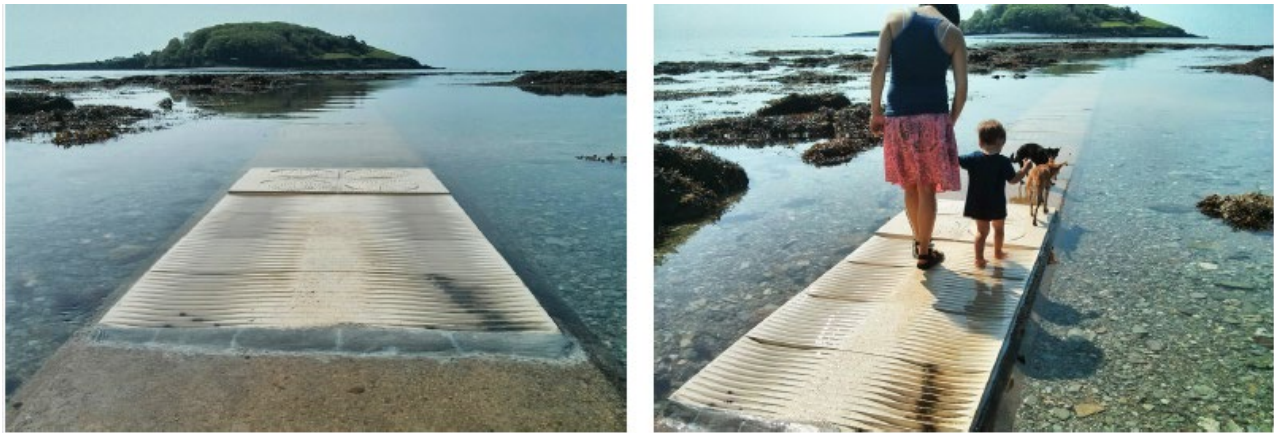
Figure 25 Eco-enhanced stormwater outfall at Hannafore beach
