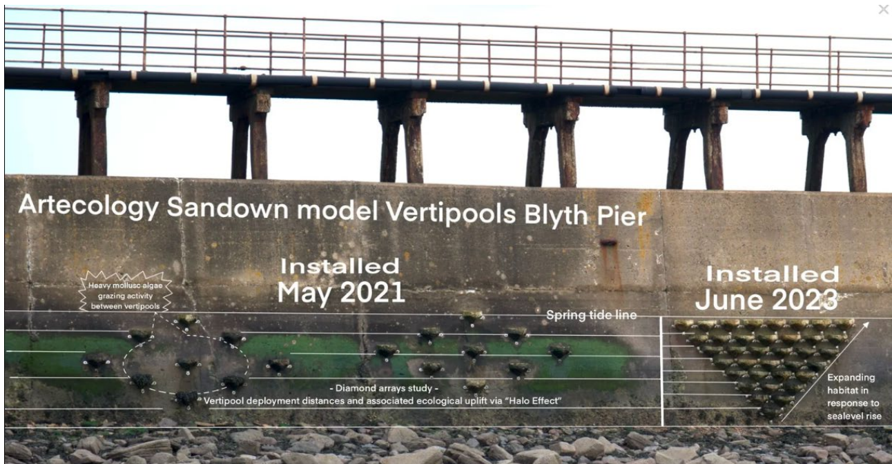
Figure 35 Blyth Pier Project array design of Vertipools installed in 2021 and 2023. Source: Artecology and Groundwork North East and Cumbria
