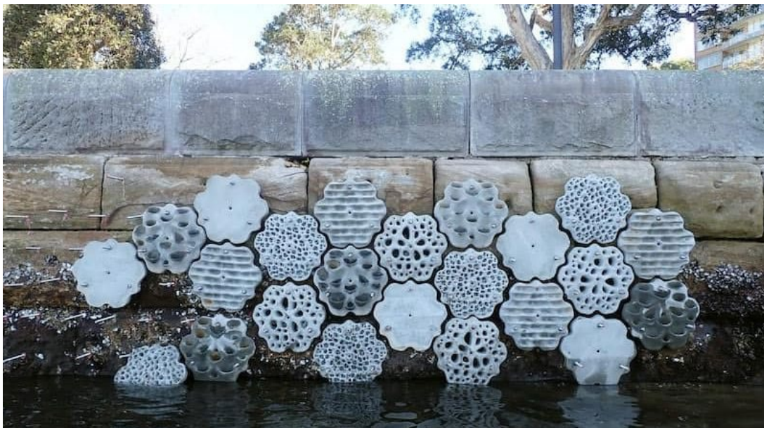
Figure 27 Living Seawalls at Sydney Harbours. [Source: https://www.sustainabilityhackers.com/living-seawalls-to-bring-new-life-to-rushcutters-bay/ ]
