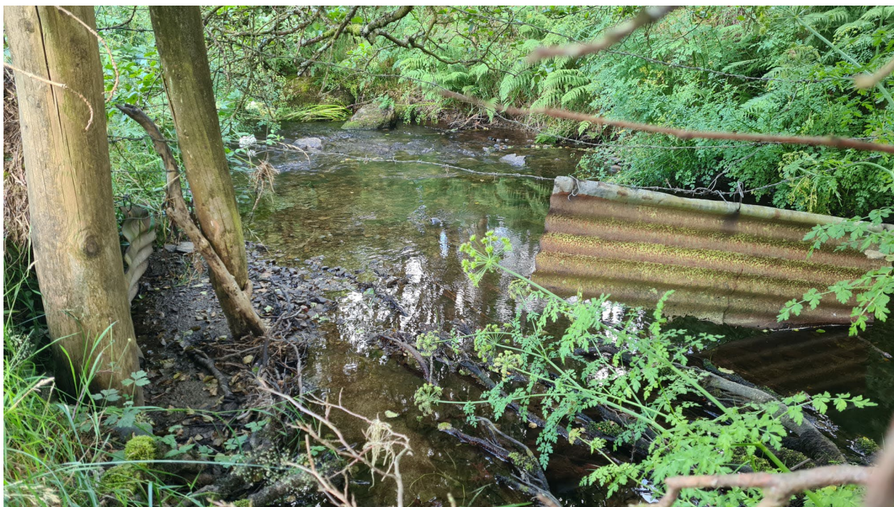
Figure 17. Photo of Nant y Dernol at the midpoint across the channel
