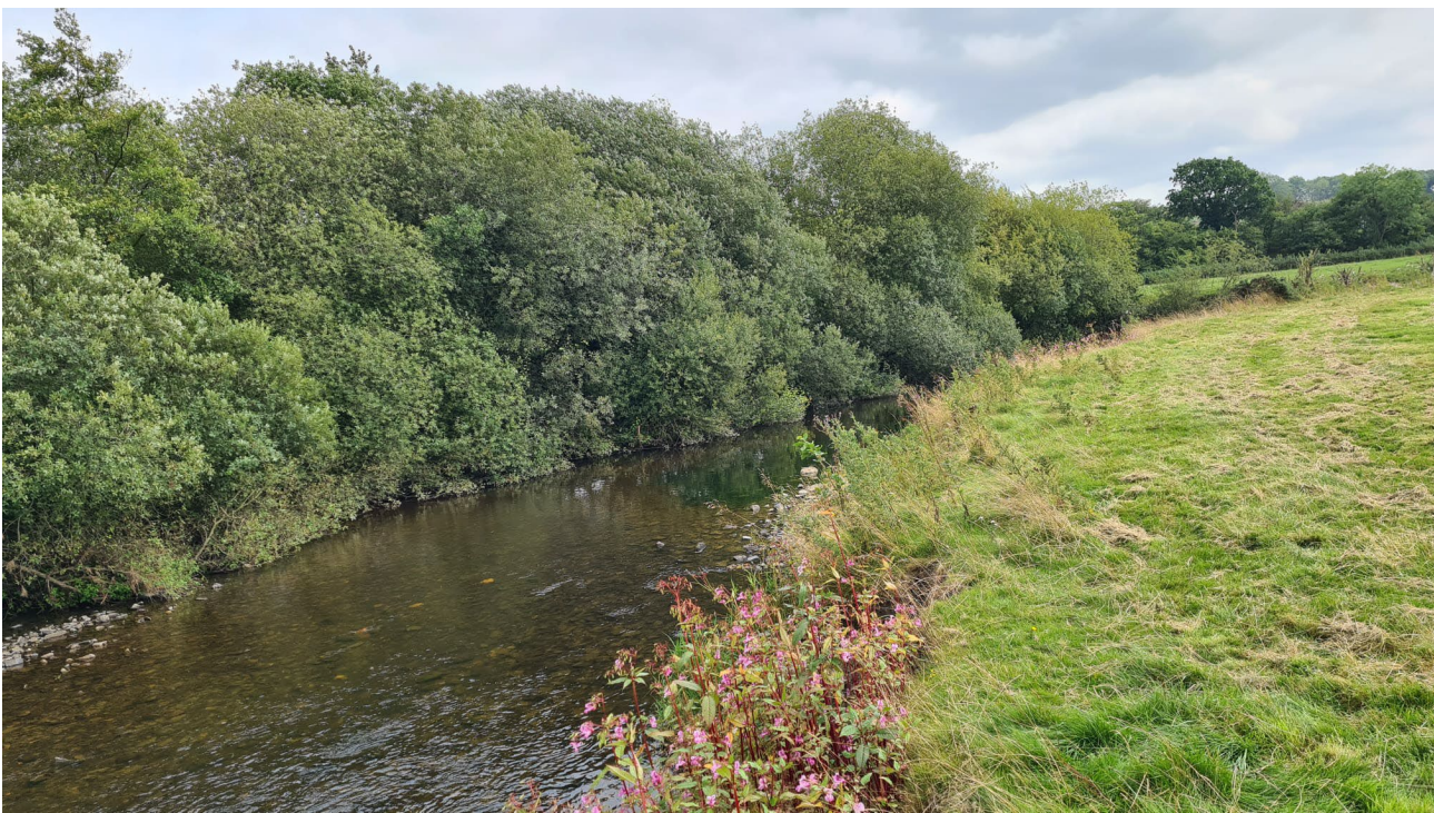
Figure 43. Photo of Ithon, d/s A485 road bridge, at the midpoint facing downstream
