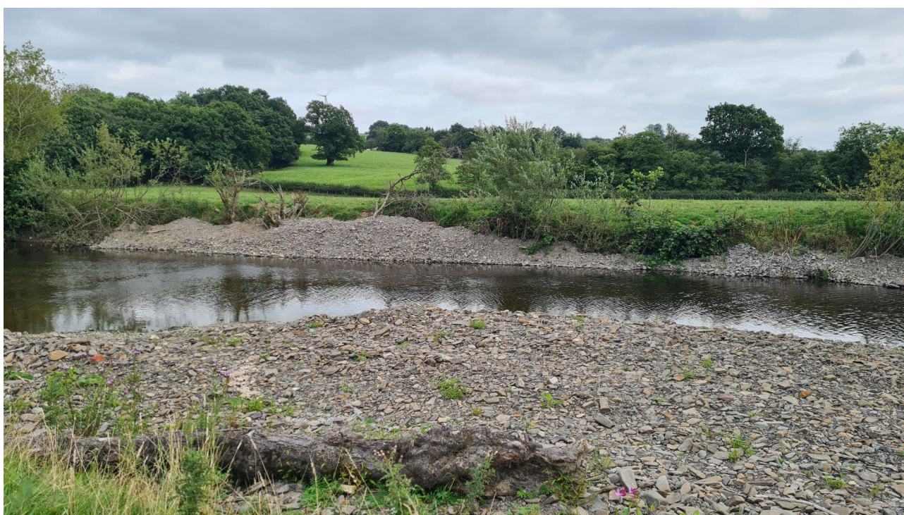
Figure 41. Photo of Ithon, d/s A485 road bridge, at the midpoint across the channel
