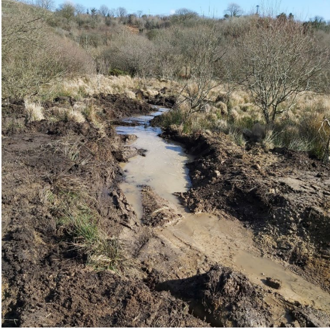
Figure 4. Waun Isaf. A newly-created stream channel carrying water away from the footpath.
