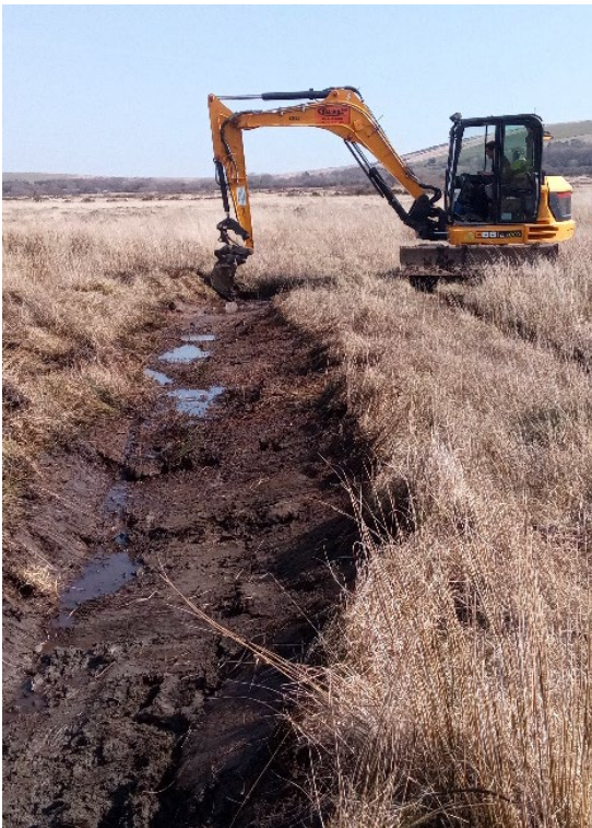
Figure 10. Dolau Isaf. Stream restoration.
