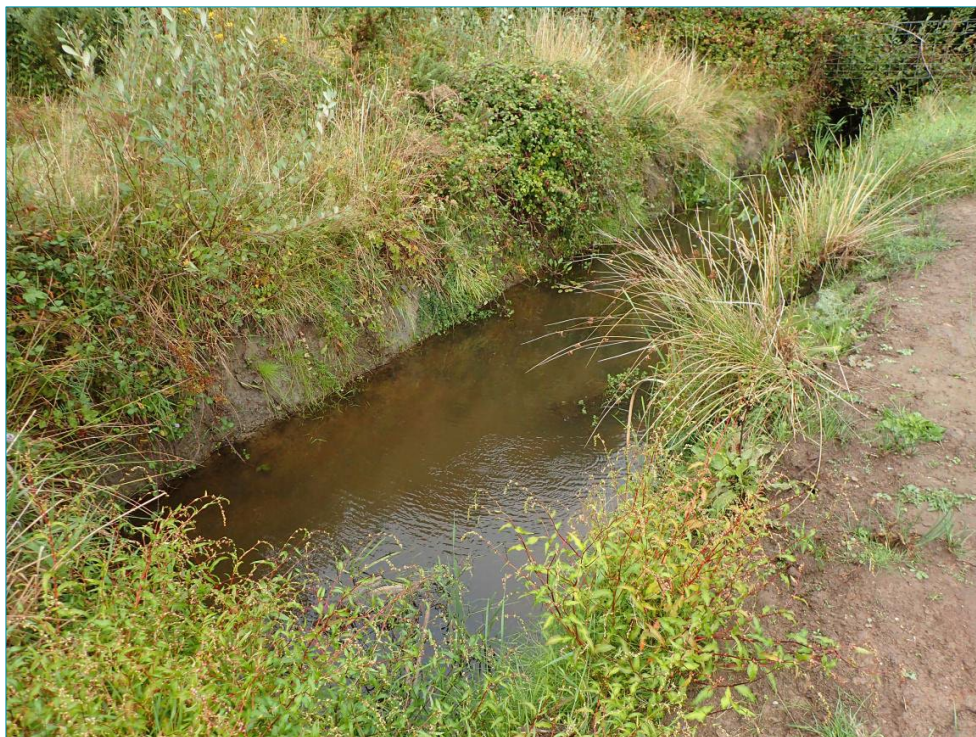
Figure 16. 'Ditch 2' showing evidence of recent clearance. September 2025.
