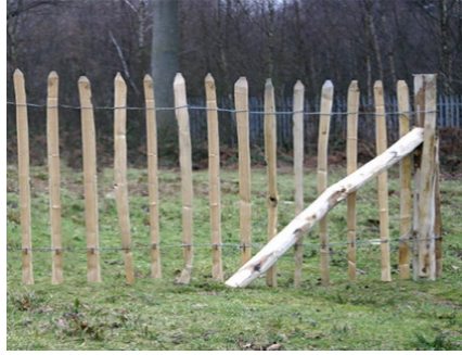
Figure 3. A simple chestnut paling fence that could be deployed to protect fish habitat in the margins.
