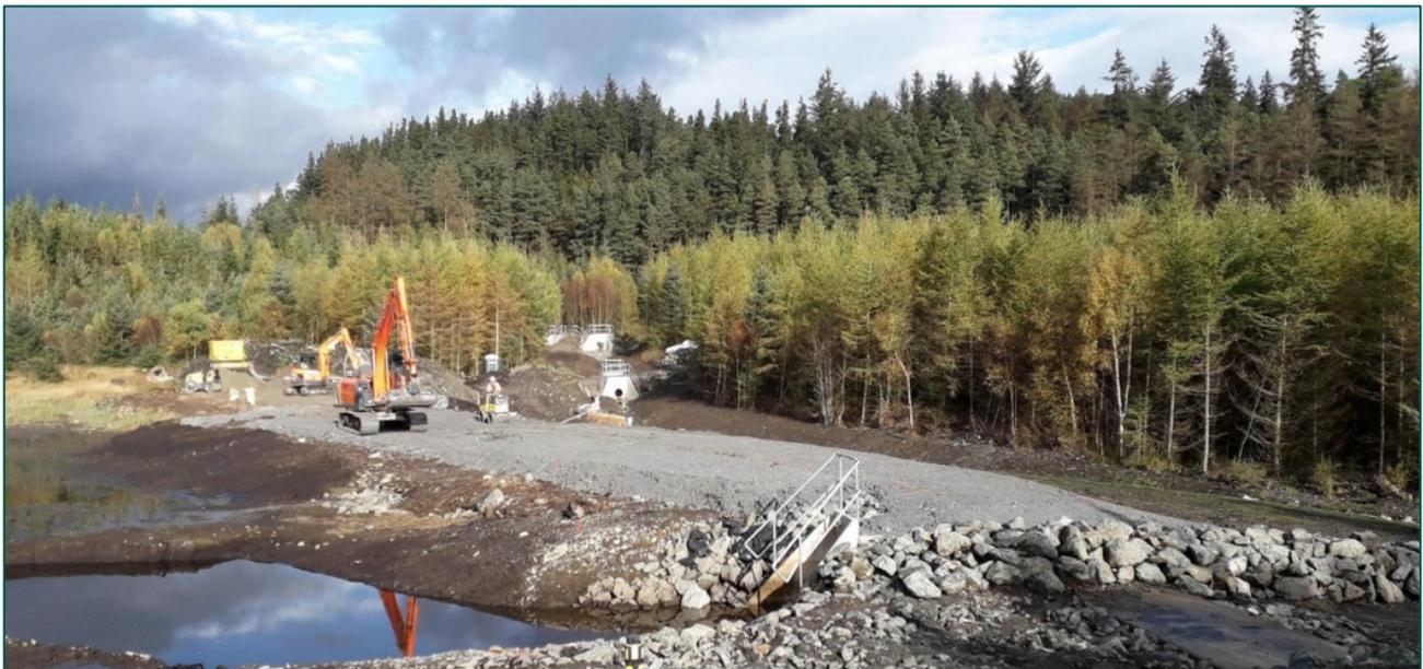
Figure 4. Completing improvements at Cyfty North, using stone blocks in preference to concrete where possible.
