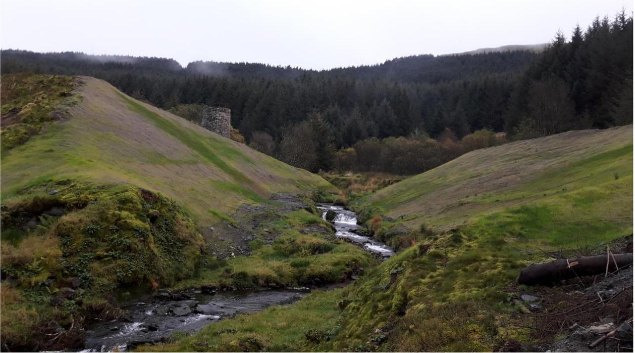
Figure 5. Looking through the notch at Llyn Llaeron which was formed to discontinue the reservoir and remove the flood risk. Additional works were undertaken to maintain heritage structures at the site.
