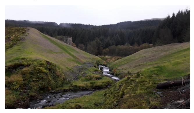
Figure 5. Looking through the notch at Llyn Llaeron which was formed to discontinue the reservoir and remove the flood risk. Additional works were undertaken to maintain heritage structures at the site.
