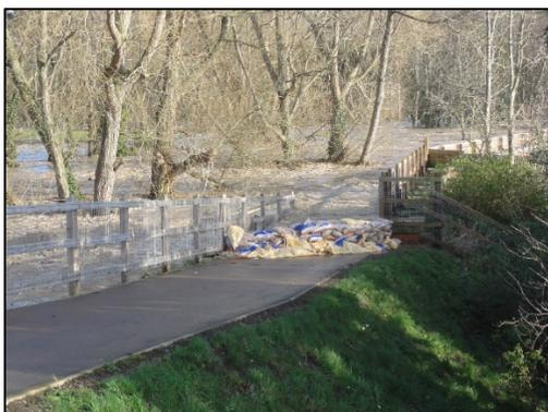
*Figure 91: River gravel deposit on Foxons Ramp (NRW, 2020)*
