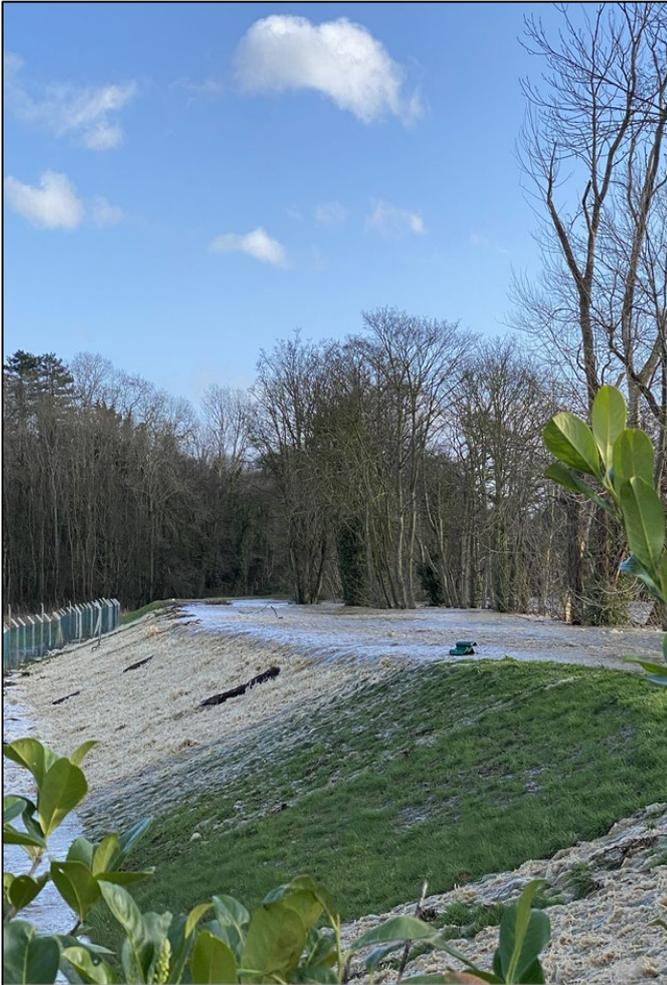
Figure 47: Localised scour caused by overtopping at the discrete low spot (NRW, 2020)
