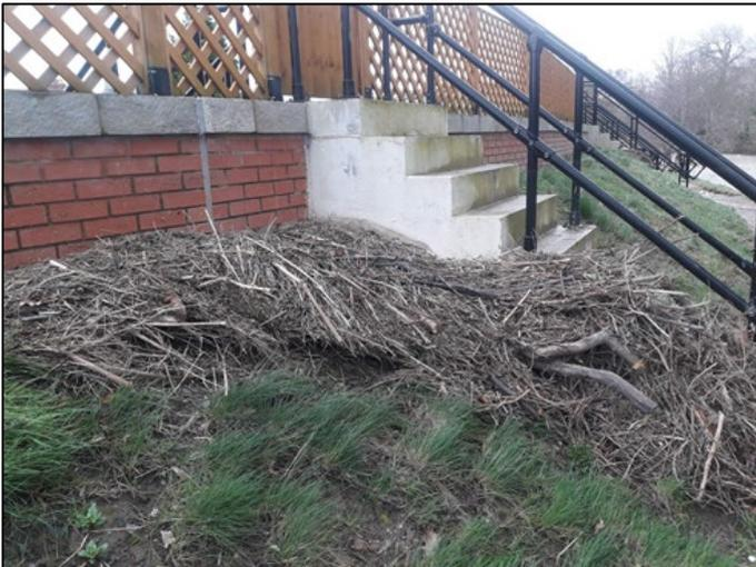
Figure 106: Wrack mark in relation to crest height common emb (NRW, 2020)
