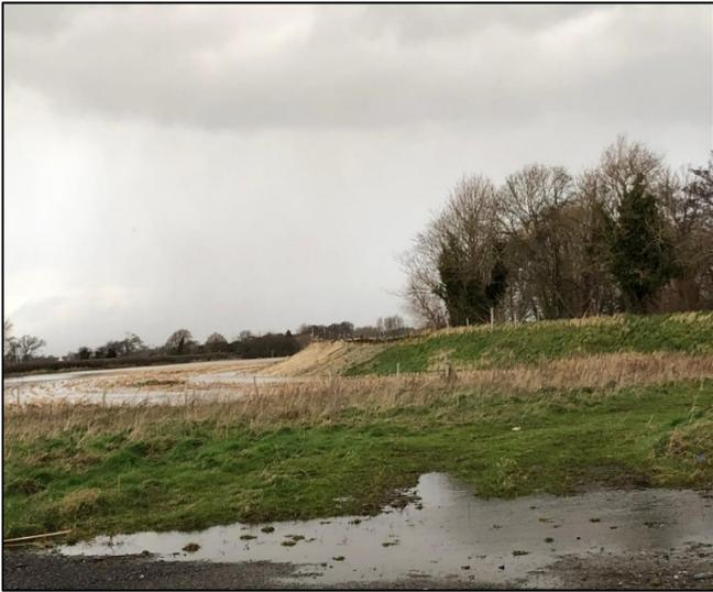
Figure 35: Phase 1 - Extensive overtopping at EMB1500412 (NRW 2020)
