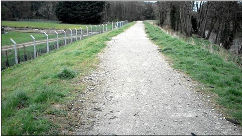
Post-event topographic survey completed by NRW confirmed that the as-built levels for Elwy right bank sewage treatment works defences were within engineering tolerances for hard and soft defences (Figure 28). There was a short length, less than 5m which was approximately 100mm lower than the design crest level.
