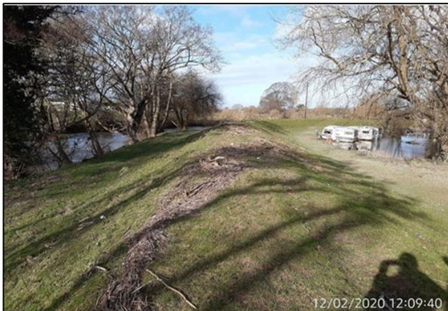
Figure 39: Wrack & debris deposits on the riverside face (NRW, 2020)
