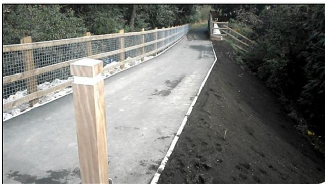
Post-event topographic survey completed by NRW confirmed that the as-built levels for Elwy left bank Roe Parc defences were within engineering tolerances for hard and soft defences (Figure 26).
