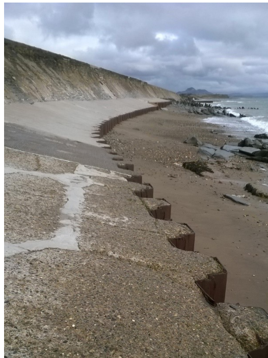
Figure 10 Coastal defences, North Wales. Photo: Heather Lewis
