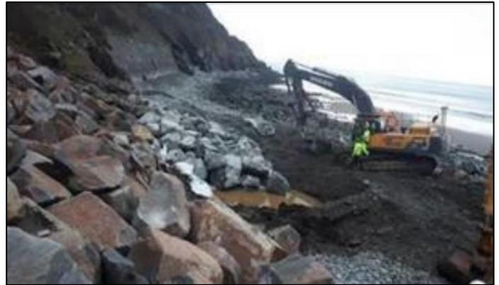
**Fig 35: Backfilling of Rock at Southern End, Friog Corner, Gwynedd**
