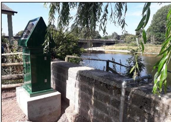
**Figure 7: A new level gauge at Glasbury, Powys. The old kiosk was situated below the 1 in 100 year flood level and powered by mains electricity. NRW relocated the kiosk so that at an appropriate level and adapted to run on solar power.**
