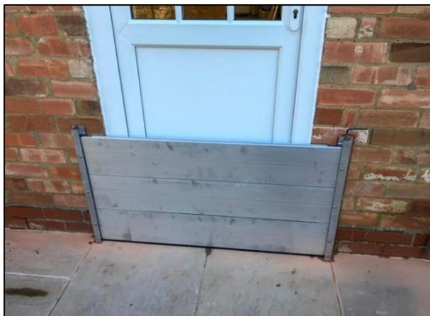
**Figure 34: example of a single door flood barrier**
