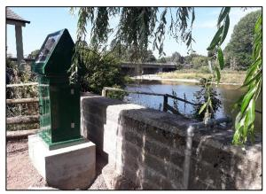
Figure 7: A new level gauge at Glasbury, Powys. The old kiosk was situated below the 1 in 100 year flood level and powered by mains electricity. NRW relocated the kiosk so that at an appropriate level and adapted to run on solar power.
