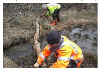
Figure 36: Work to install leaky dams at Solva
