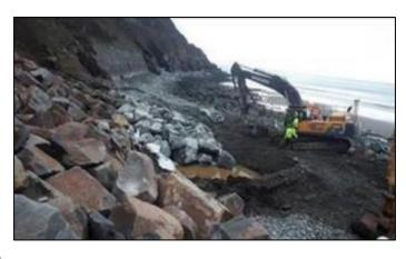
Fig 35: Backfilling of Rock at Southern End, Friog Corner, Gwynedd
