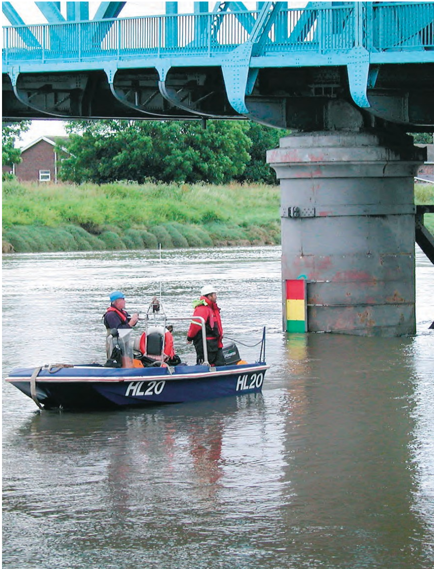
Figure 3 Photograph of a safety boat in attendance during harbour works at the Queensferry Blue Bridge.
