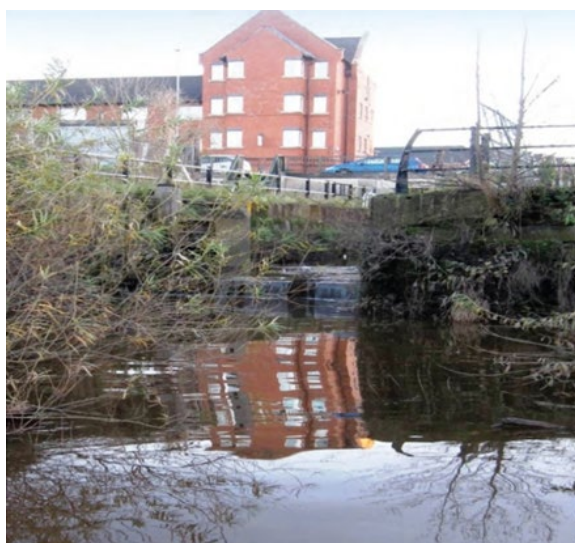
Figure 17 Lock gates at the entrance to the Shropshire Union Canal.
