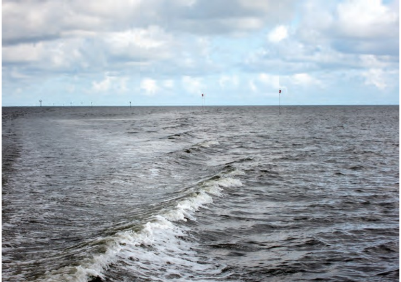
Figure 6 North Training Wall light tower and piles looking seaward over submerged wall.
