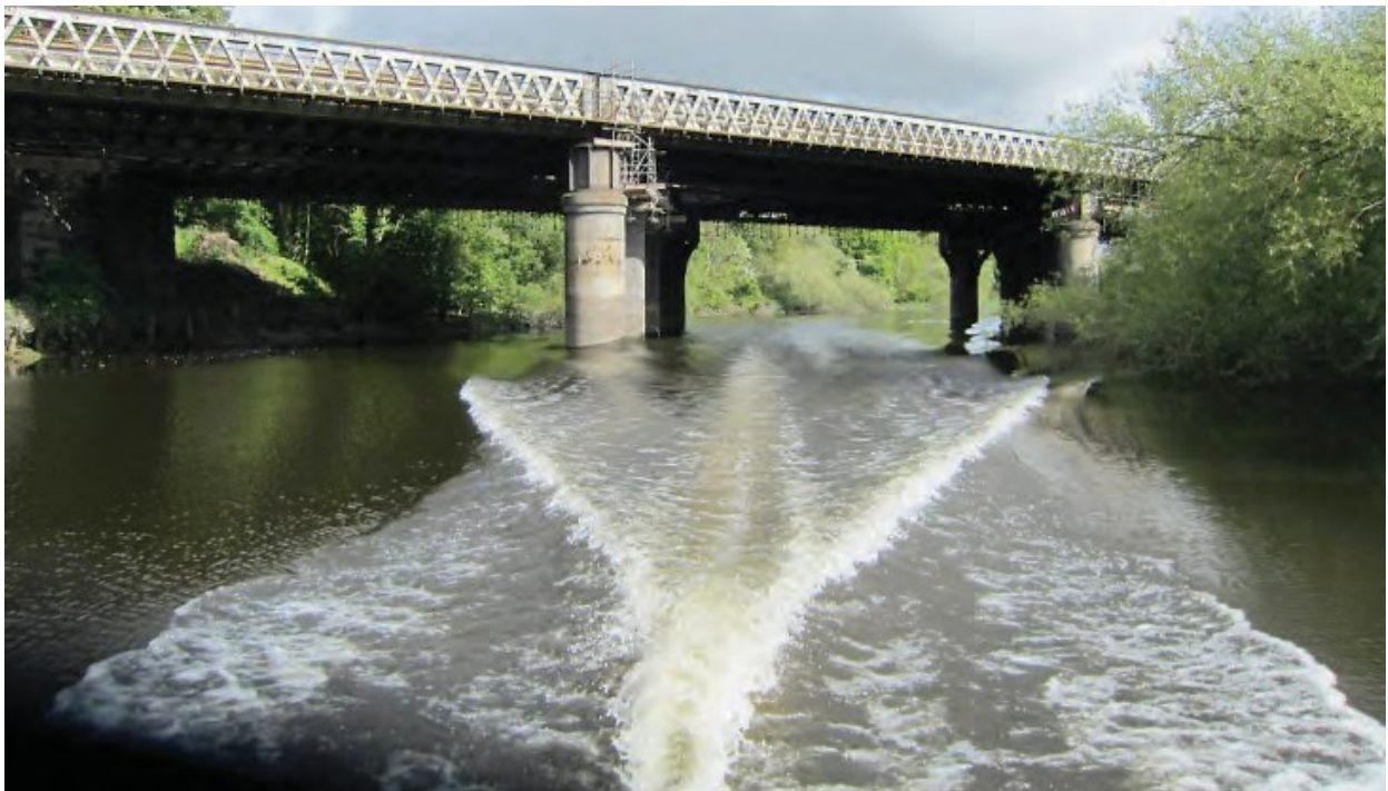
Figure 18 Rail bridge at Wilcox Point marking the upstream limit of the Dee Conservancy.
