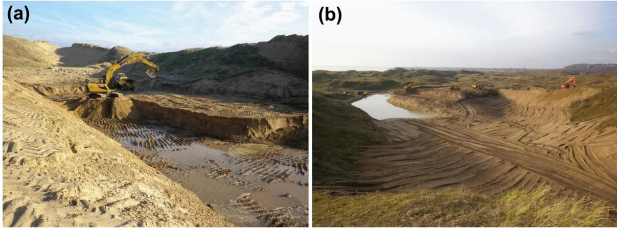
**Figure 30.** Merthyr Mawr Phase 1, December 2012: (a) Sand excavation in progress to create an artificial slack; (b) work to create slack and extend / raise dune arms near completion (photographs by D. Ludlow, NRW)
