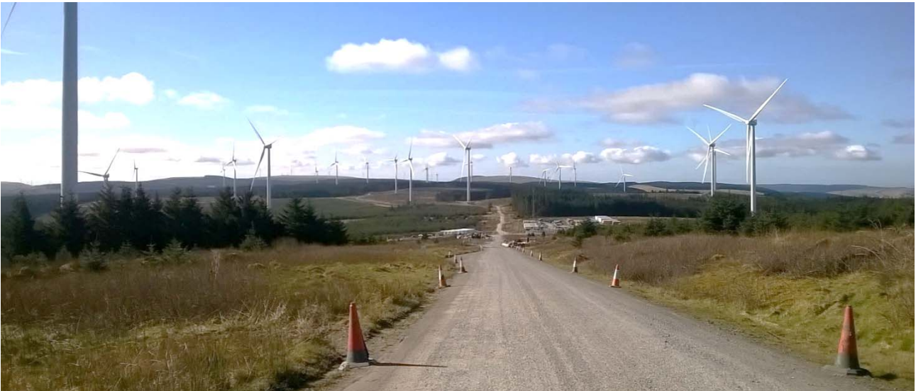
Figure 16: Rolling upland wind turbine landscape at Pen-y-Cymoedd. Areas identified in TAN 8 Strategic Search Areas for wind farms are typically like this: extensive, sparsely populated upland plateaux, dominated by impoverished moorland and/or conifer plantation and a general absence of nature conservation, landscape or heritage designations. The wind turbines and their access tracks are fitted into a landscape already managed for extensive plantation forestry and moorland.
