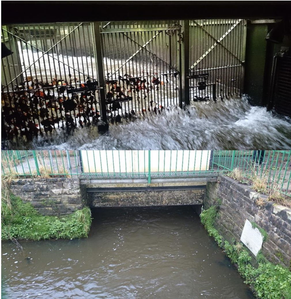
Figure 17. Upstream gate from inside the fish trap preventing fish from continuing upstream (top). Downstream entrance to the fish trap directly above the fish ladder (bottom).
