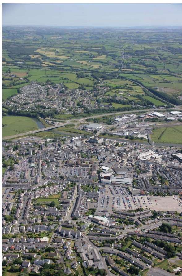
Carmarthen: © Crown Copyright: RCAHMW
