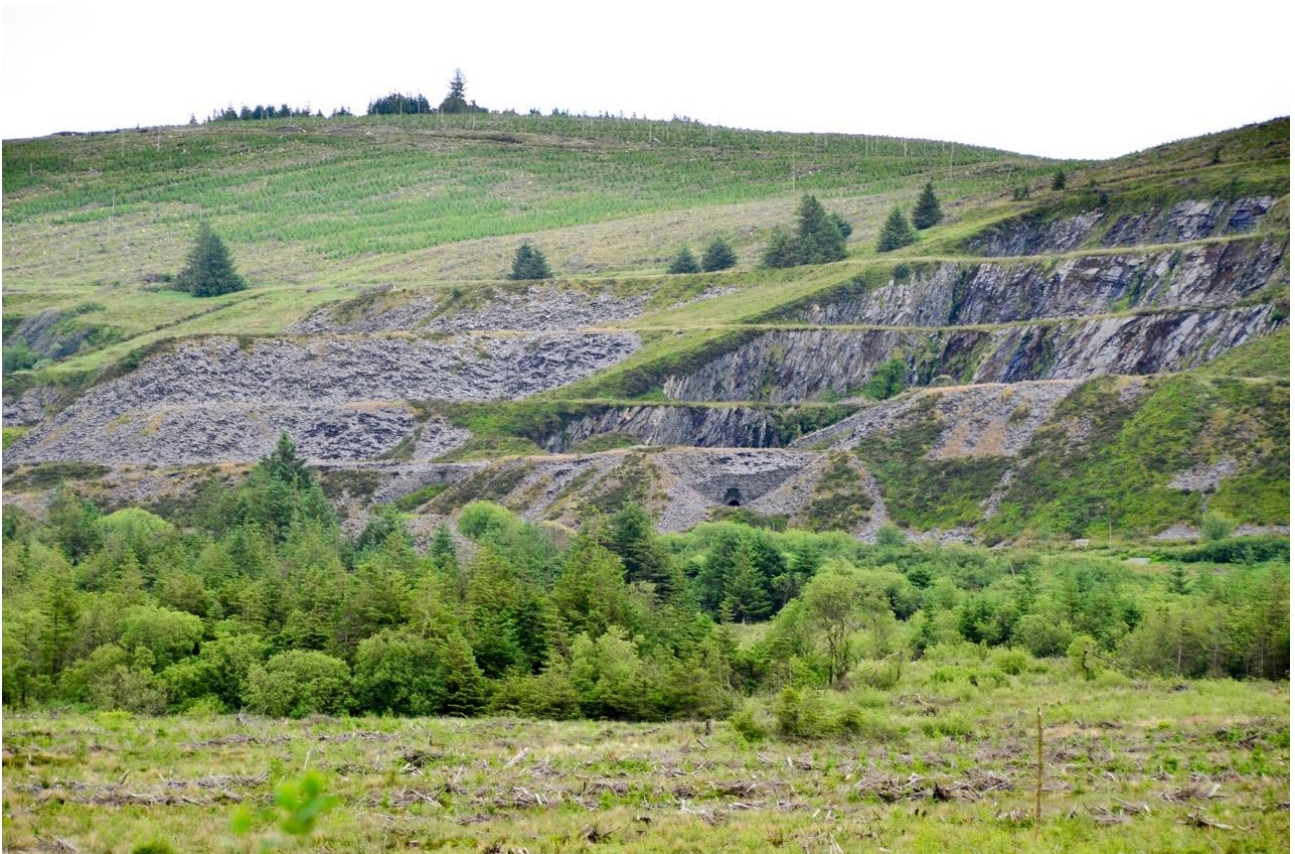
Rosebush - remains of old slate quarries and new coniferous plantation © John Briggs
