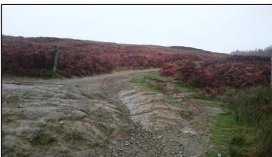
*Exposed bedrock re-graded to provide a more accessible surface on byway LC294. Some sections were difficult to pass even in 4x4 vehicles before work was undertaken*
