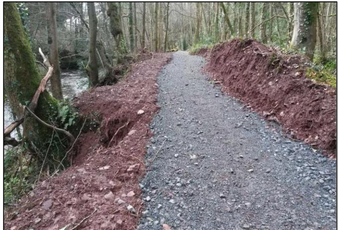
**After** – The pathway is now 1200mm wide and the path has been moved away from the drops, the pathway which was originally undulating has now been levelled to allow easier access to this area within Priory Groves.
