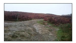
Exposed bedrock re-graded to provide a more accessible surface on byway LC294. Some 9 sections were difficult to pass even in 4x4 vehicles before work was undertaken
