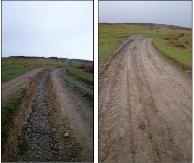
Deep rut on byway LC294 caused by a combination of motor vehicle use and water damage before and after repair.
