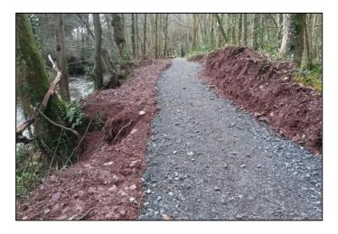
After – The pathway is now 1200mm wide and the path has been moved away from the drops, the pathway which was originally undulating has now been levelled to allow easier access to this area within Priory Groves.
