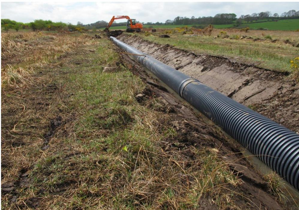
**Figure 14.** Infill of ditch section A-B and burial of the bypass pipe at Cors Bodeilio NNR, 8 May 2013. The peat infill visible in the distance was sourced from peat cutting areas in compartment CB1NE. Photo looking SW with Ynys on left. Original file number IMG\_8110.
