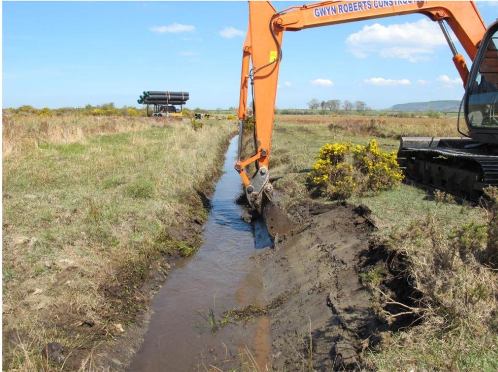
**Figure 13.** Cleaning of ditch section A-B to create a graded bed for the bypass pipe. Sections of bypass pipe can be seen in the distance tied onto a steel cage mounted on a tracked dumper. Image taken 7 May 2013, looking NE from close to point A. Original image number IMG\_8085.
