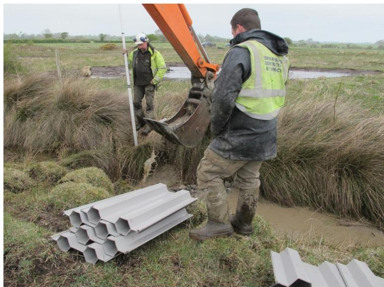
Four dams were installed (all on 10 May 2013), with the crest of the first (Dam 1 – see Table 7) set under laser levelling control to a level just beneath that of the top of the bypass pipe outlet. Relevant height and location details are given in Table 7.
