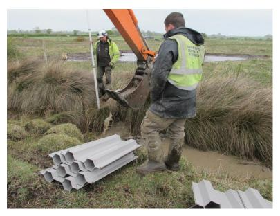
Four dams were installed (all on 10 May 2013), with the crest of the first (Dam 1 – see Table 7) set under laser levelling control to a level just beneath that of the top of the bypass pipe outlet. Relevant height and location details are given in Table 7.
