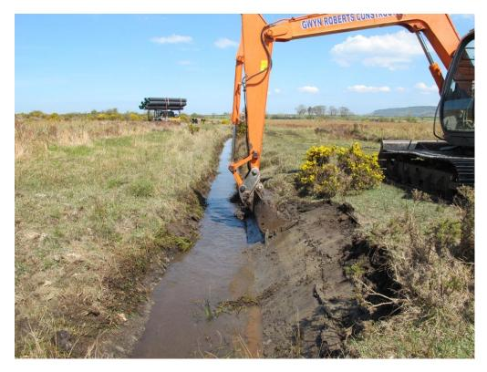
**Figure 13**. Cleaning of ditch section A-B to create a graded bed for the bypass pipe. Sections of bypass pipe can be seen in the distance tied onto a steel cage mounted on a tracked dumper. Image taken 7 May 2013, looking NE from close to point A. Original image number IMG\_8085.
