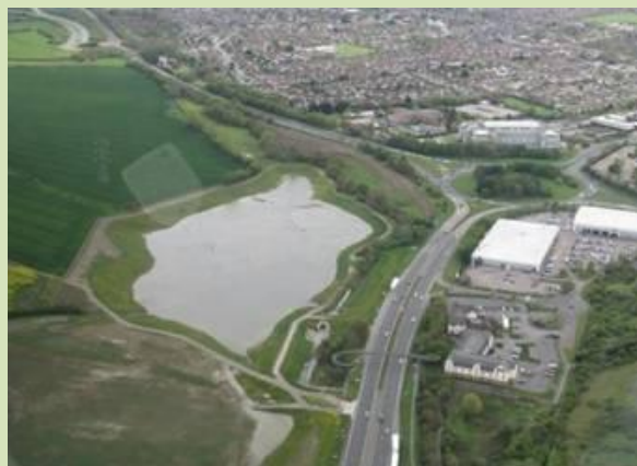
Horsbere Brook flood defence scheme, Gloucester
