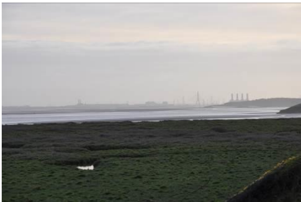
Deeside Power Station
