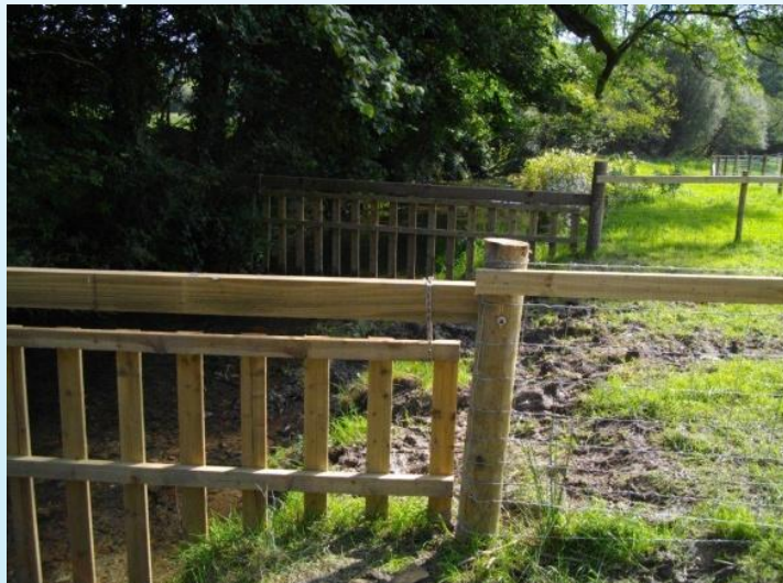
Fencing work on the Cerdin. Photo credit: John Morris
