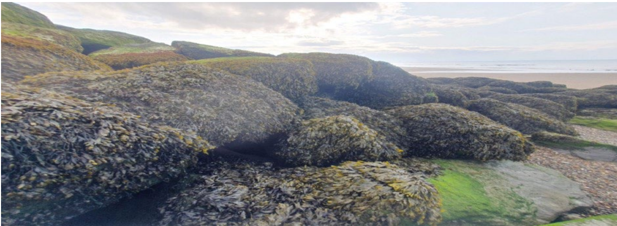
Figure 11. New artificial coastal defence structure at Rhyl with Superabundant F. spiralis in 2024
