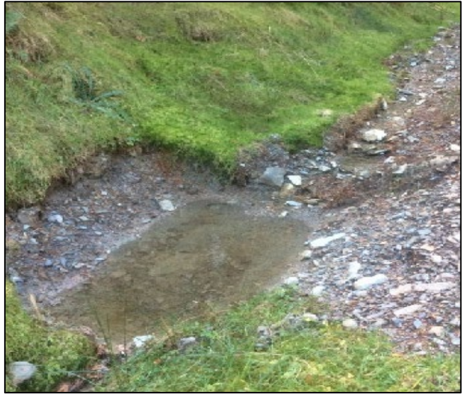
Figure 6-2: Catch pit. NGR: SN 87733 80263
