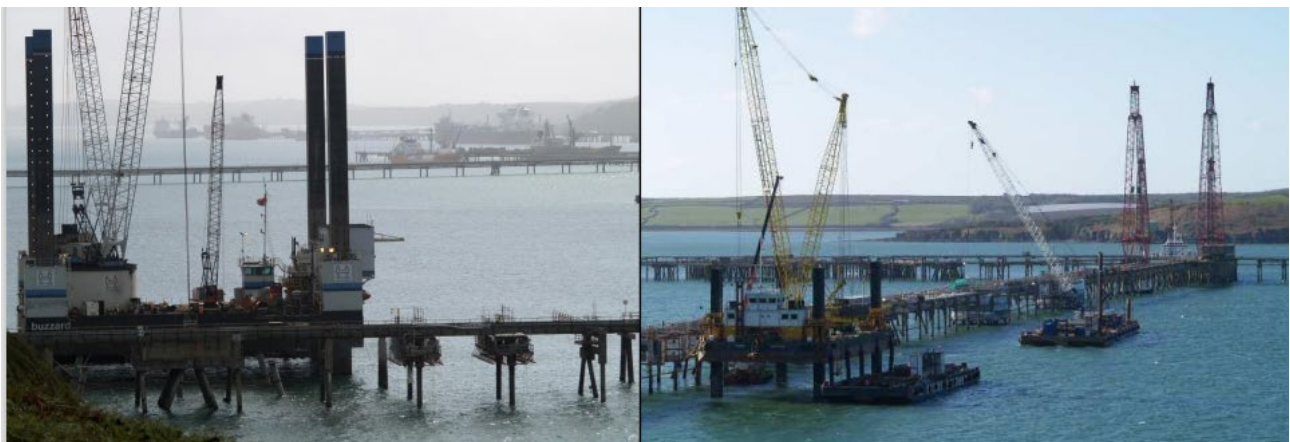
Figure 13: Jack-up barges. Photo: M. Camplin (April, 2006).
