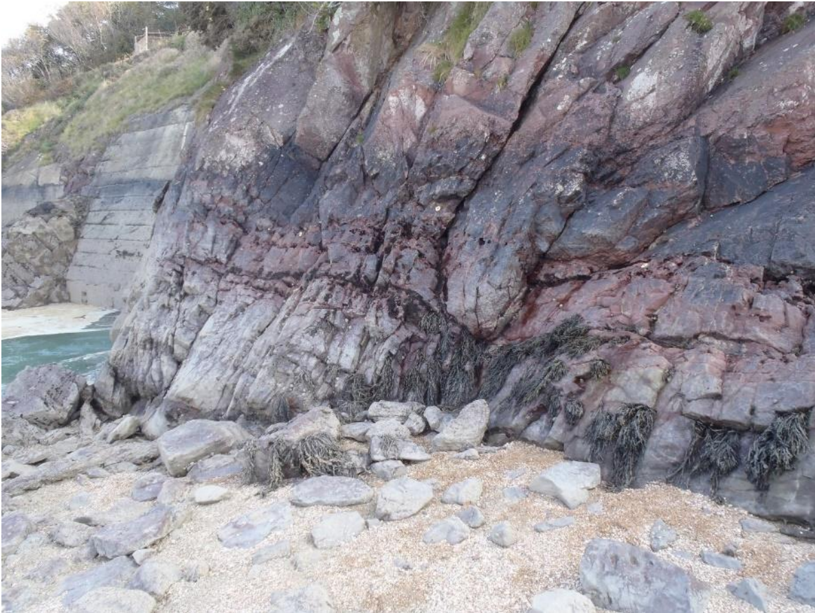
Figure 14 Images of Upper Shore Pembroke Power Station Site (Upper image: 2014, Lower image: 2021)
