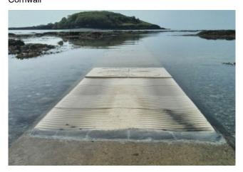
Figure 5 Technique 4 Cast-in textured, grooved and creviced concrete surfaces
