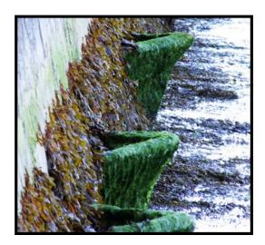
Figure 7 Technique 6 – Bolt on precast vertical pools
