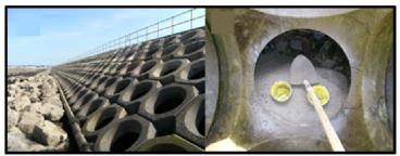
Figure 4 Technique 3 cast-in rockpools [Source: Firth et al.,2014]
