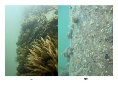
Figure 16 (a) ecological jackets and (b) control - fiberglass jacket. Both are 14 months post-deployment.
