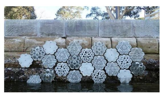
Figure 12 Living Seawalls at Sydney Harbours. [Source:https://www.sustainabilityhackers.com/living-seawalls-to-bring-new-life-to-rushcutters-bay/]
