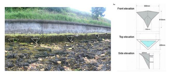
Figure 14 Location of the Vertipools on the seawall (left) and dimensions of the Vertipools (right) [Source: From Hall et al. (2019)]
