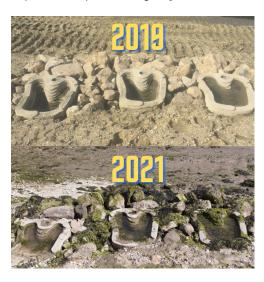
Figure 9 Technique 8 – Drop-in prefabricated units
