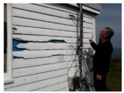
In 2019 the old Coastguard lookout hut on the Deer Park was refurbished as the outer timber "skin" had rotted guite badly. This entailed the temporary removal of the NRW automatic weather station by MCZ staff and its replacement following the building work.
