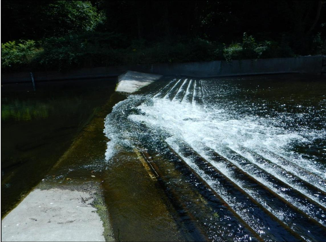
*Low Cost Baffle (LCB) solution at Resolven gauging weir – River Neath 2017*
