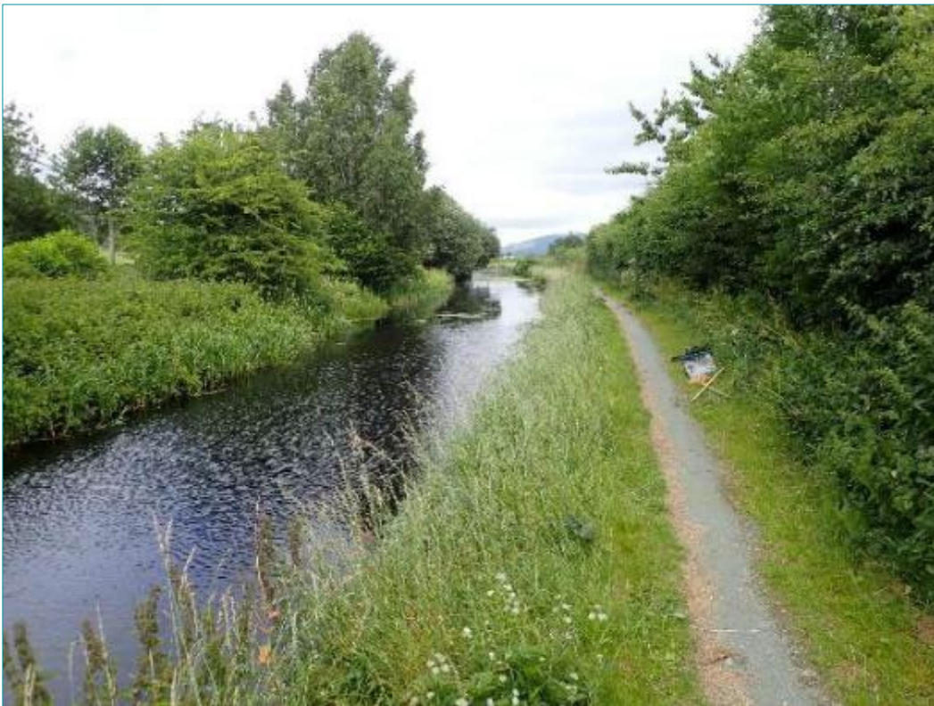
Photograph 22. Brithdir Lock. View is looking northeast. 24 th June 2025.
