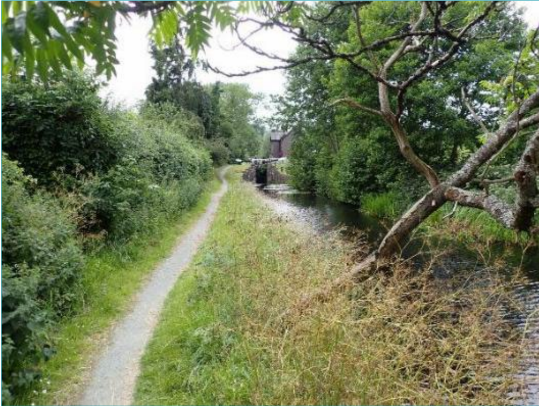
Photograph 21. Brithdir Lock. View is looking southwest. 24 th June 2025.
