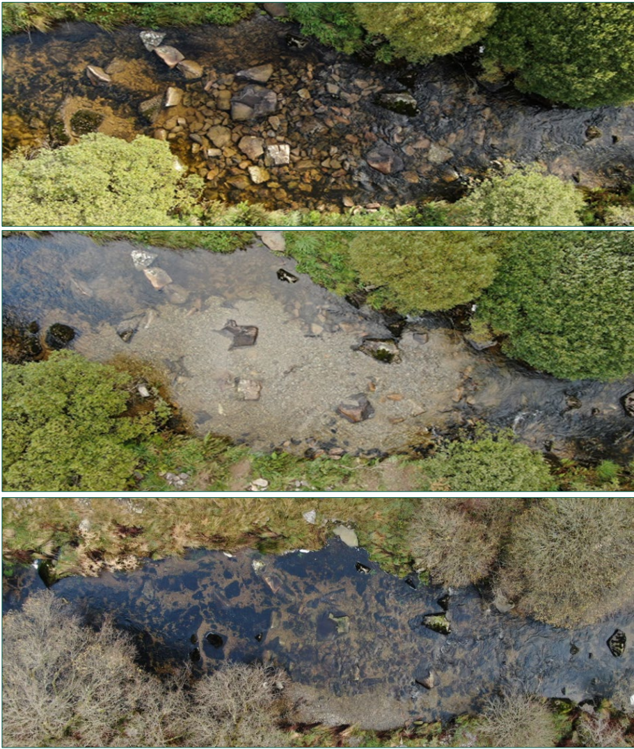
Figures 51, 52 & 53. Stages in habitat restoration on the Afon Eden. Top: immediately following boulder reintroduction, May 2022. Middle: following gravel reintroduction. Bottom: December 2022, following gravel redistribution by flood flows. Additional boulders trap gravel around them, maintaining stable well-oxygenated habitat for juveniles.
