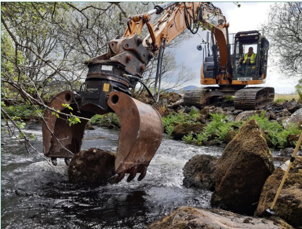
Figure 50. Digger replacing boulders to restore habitat in a pearl mussel river.
