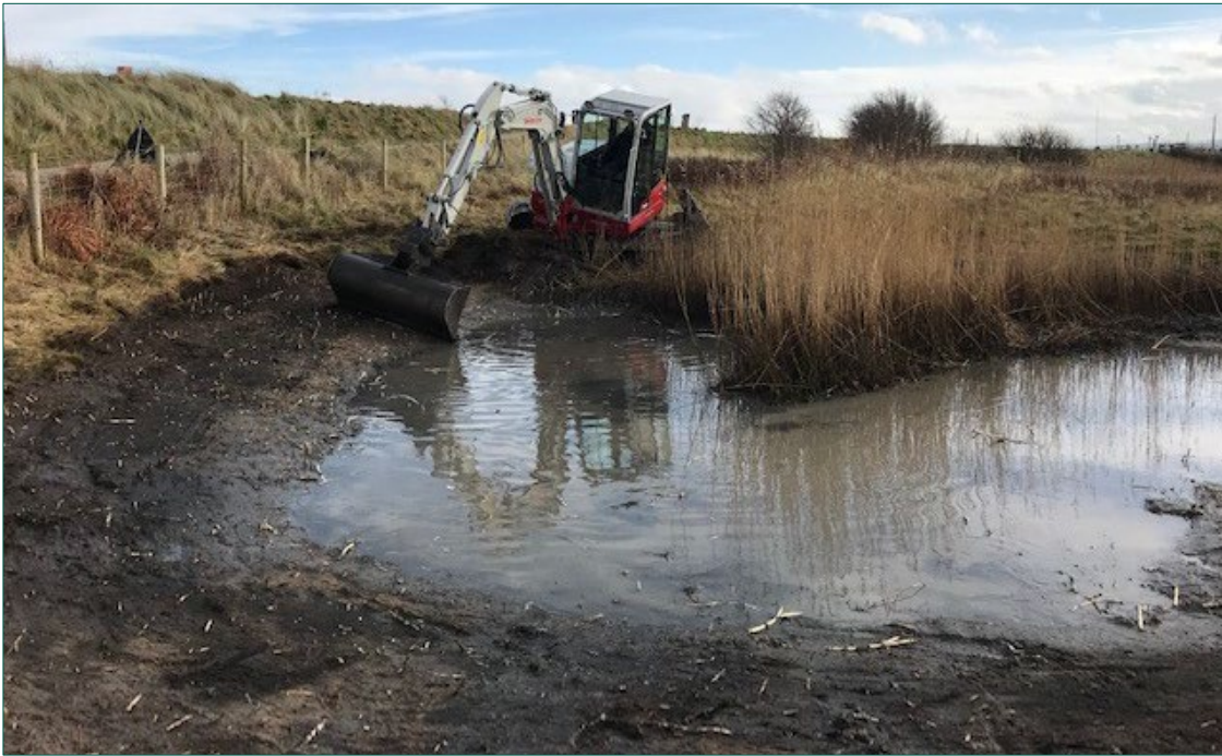
Figure 54. Re-profiling a pool occupied by Natterjack Toad Epidalea calamita © Kim Norman
